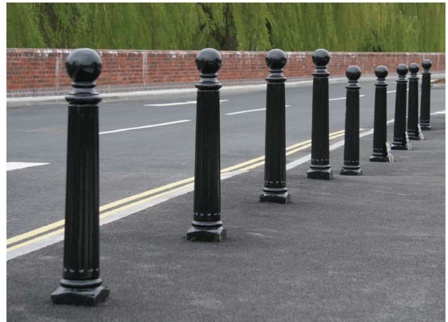
Ferrocast root fixed and removable Seaham bollards, Bewdley, Worcestershire.
