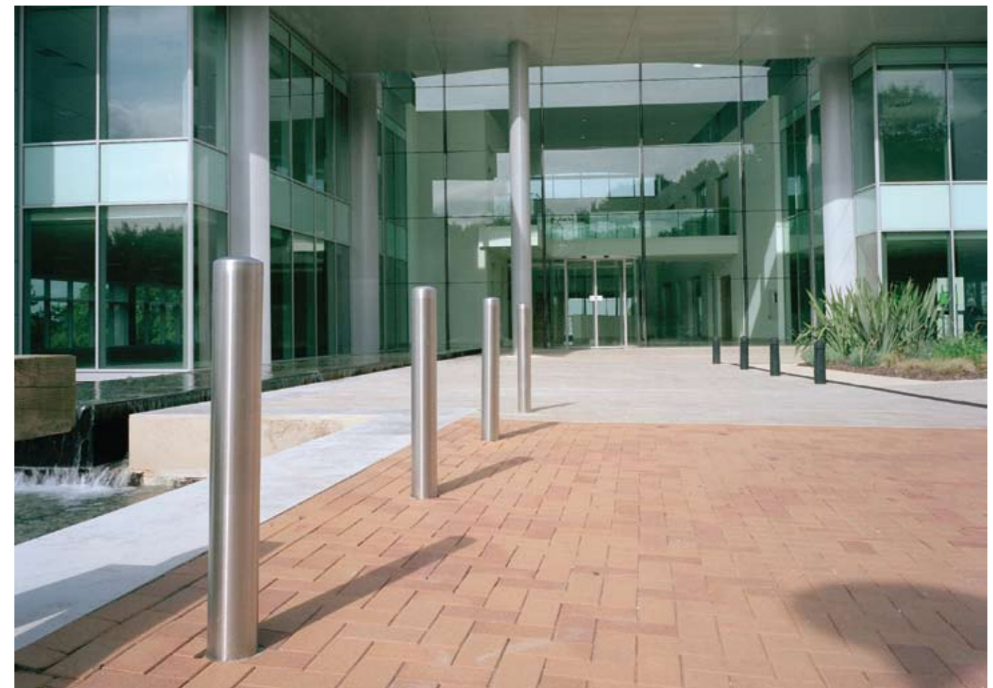
RS 001 Stainless Steel Bollards, Basingstoke
