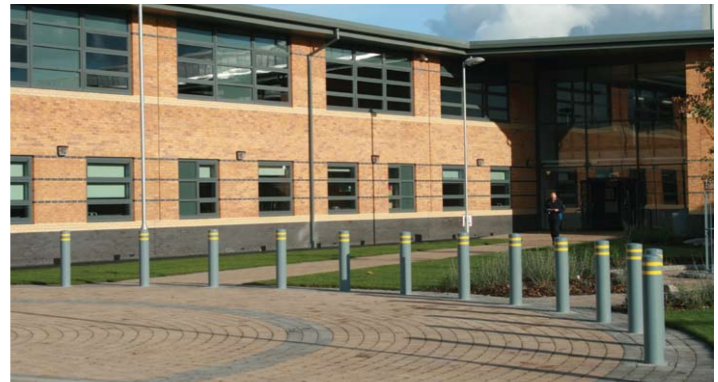
RB 111 Steel Bollards with yellow banding on Tegula block paving in Traditional and Pennant Grey, Harrop Fold High School, Salford
